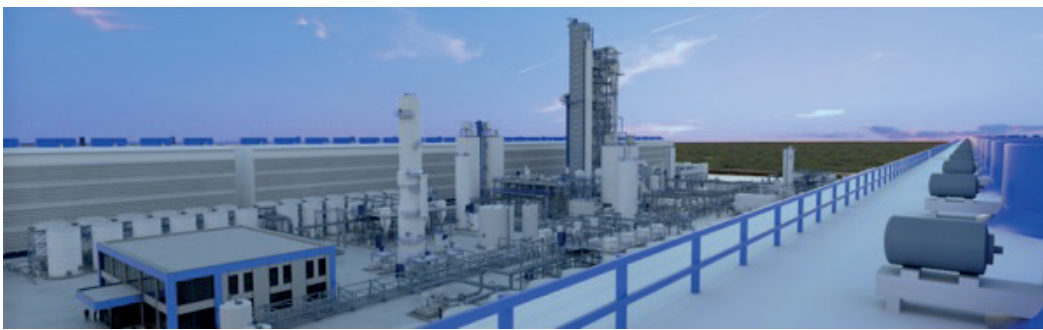
Figure 3: Artist's rendering of STRATOS, currently under construction in West Texas by 1PointFive, deploying Carbon Engineering's DAC technology.
